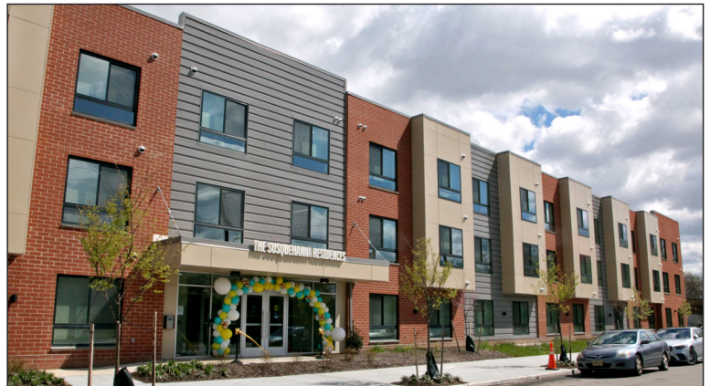
The Susquehanna Residences is a 78-unit senior building in Strawberry Mansion.
