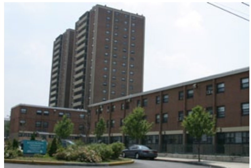
PHA will demolish two-family high-rises and 18 low-rise buildings at Blumberg as part of the agency’s comprehensive transformation plan for the neighborhood.
