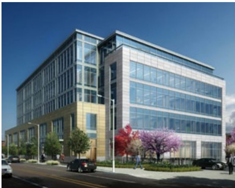
The PHA board has approved a $45 million contract for the construction of the agency's new headquarters building on Ridge Avenue. The new location will allow for the consolidation of several housing authority offices at one location.
