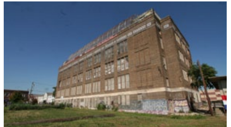
Graffiti classrooms inside the historic Spring Garden School will be rehabilitated into apartments for veterans and seniors. The construction work at the site represents the final segment of redevelopment of the Richard Allen Homes.
