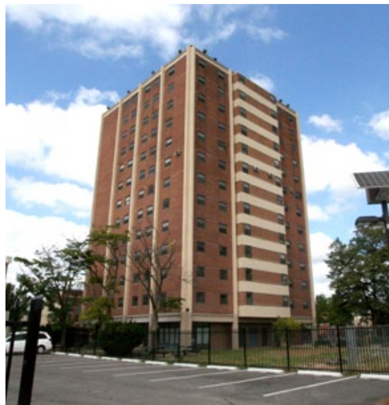
PHA expects the modernization of the Blumberg senior tower to be completed next fall. It is adjacent to Blumberg Phase I on 24th Street.
