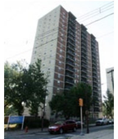
HUD has awarded PHA a $250,000 emergency safety and security grant for the Fairhill Apartments in North Philadelphia. PHA intends to use the grant funds, in combination with $641,800 in existing funds, to install a comprehensive network of security cameras that will be strategically located throughout the development.
