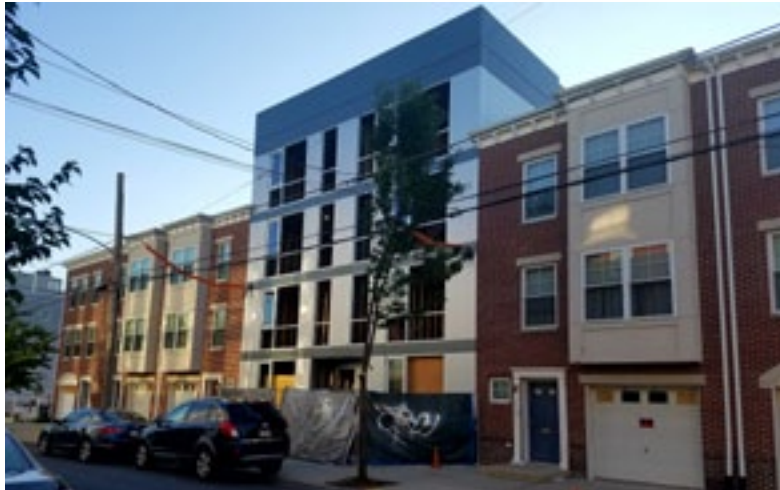
This private 4-story development in the 1400 block of north 7th Street typifies the investment that PHA and APM, its partner in the Ludlow infill development, had hoped to attract to the neighborhood ten years ago.
