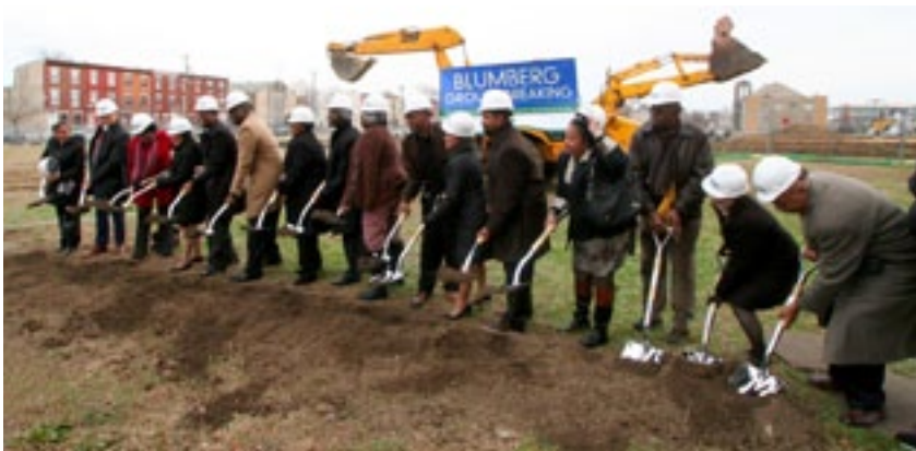
The rehab of the Blumberg Senior Tower and street construction project formally began with a groundbreaking ceremony just before Christmas. PHA is investing over $36 million for this phase of the Choice Neighborhood Transformation Plan for Sharswood/Blumberg.
