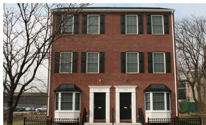
Construction will begin in April for more homes like these at Ludlow in North Philadelphia.
