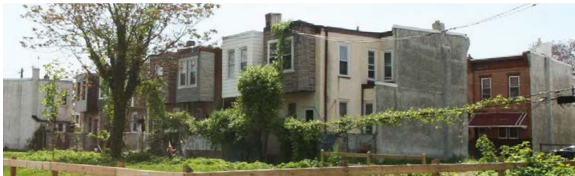
The 2800 block of Oakdale Street at the northern edge of the Strawberry Mansion neighborhood will be redeveloped by PHA and contain nine units. This part of the development is located behind the Widener Library on Lehigh Avenue.
