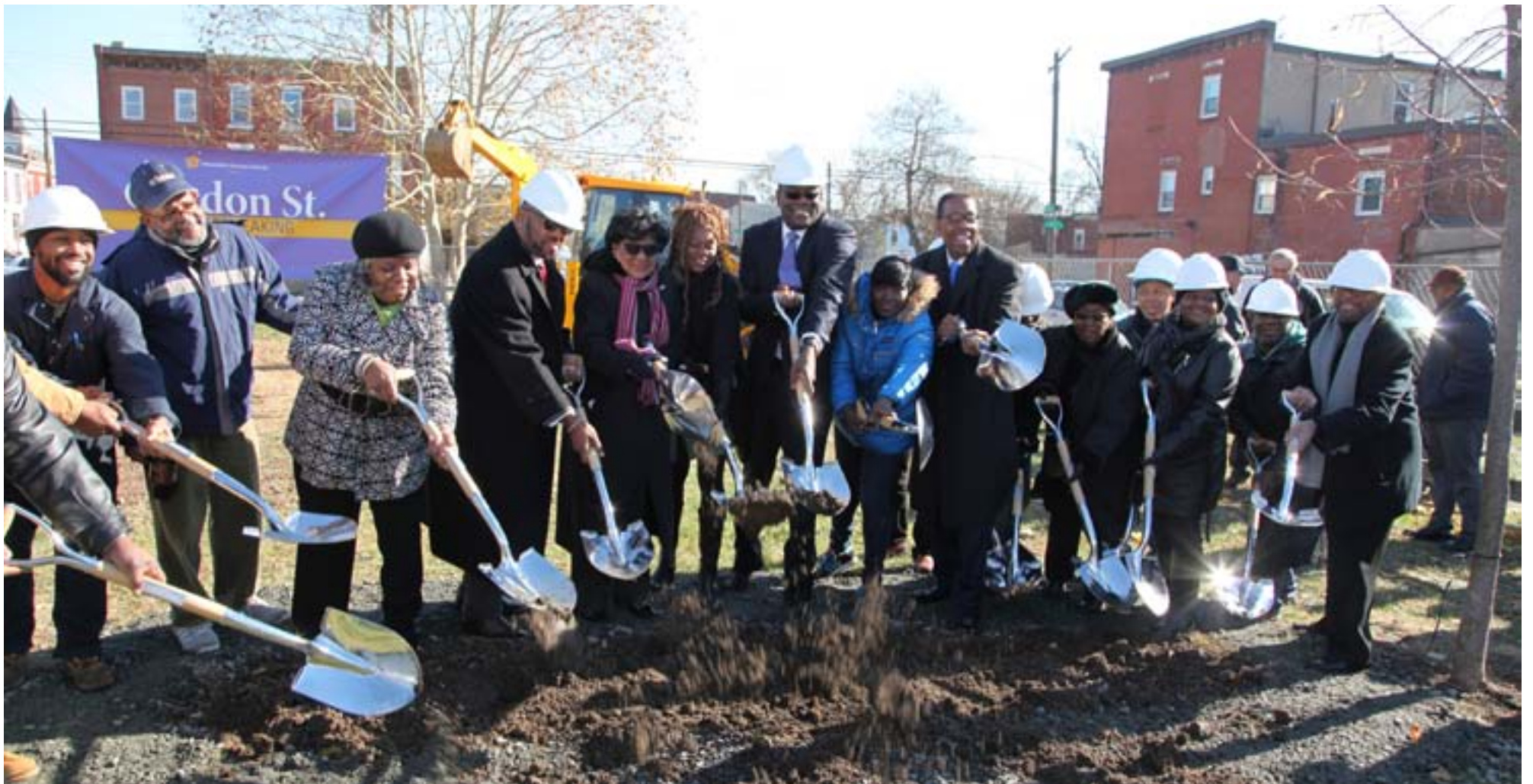
Formal groundbreaking took place in the Strawberry Mansion neighborhood for the Gordon Street Apartments. PHA President and CEO Kelvin A. Jeremiah (center) and City Council President Darrell Clarke (right) were joined by PHA Commissioners Asia Coney and Ethel Wise, City Councilwoman Jannie Blackwell, Kevin Upshur of the Strawberry Mansion Learning Center, Gordon Street Block Captain Thomas Willis, and other community members.
