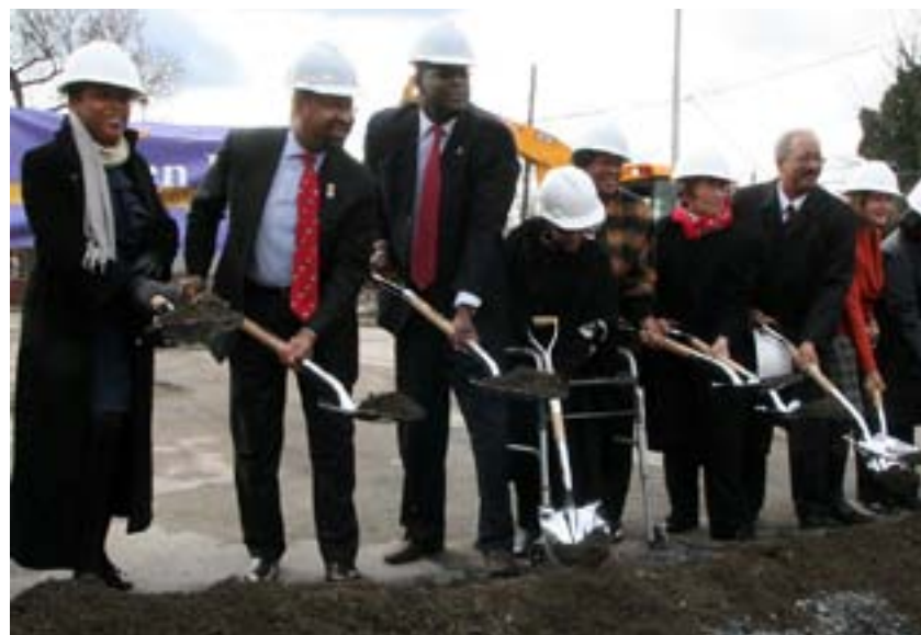
The Philadelphia Housing Authority broke ground for the new Queen Lane Apartments in historic Germantown. The new $22 million development will be constructed on the site of the 1950s high-rise that was imploded in September. Show here (l-r) are Councilwoman Cindy Bass, Mayor Michael A. Nutter, PHA President & CEO Kelvin A. Jeremiah, Queen Lane Resident Council President Corliss Gray, State Rep. Rosita Youngblood, PHA Commissioner Bonnie Camarda, Congressman Chaka Fattah, and Jane Vincent, Regional Administrator for HUD.
